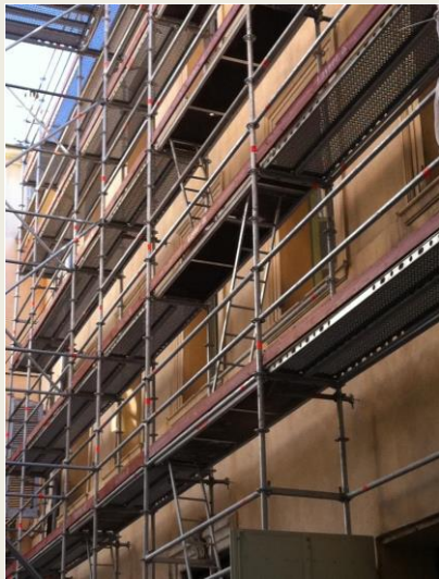
Scaffolding spans the façade
