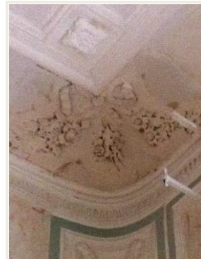
Classroom ceiling detail, 8 rue de Littera
