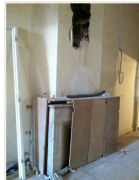
Classroom 17th century marble fireplace under protective wraps, 8 rue de Littera
